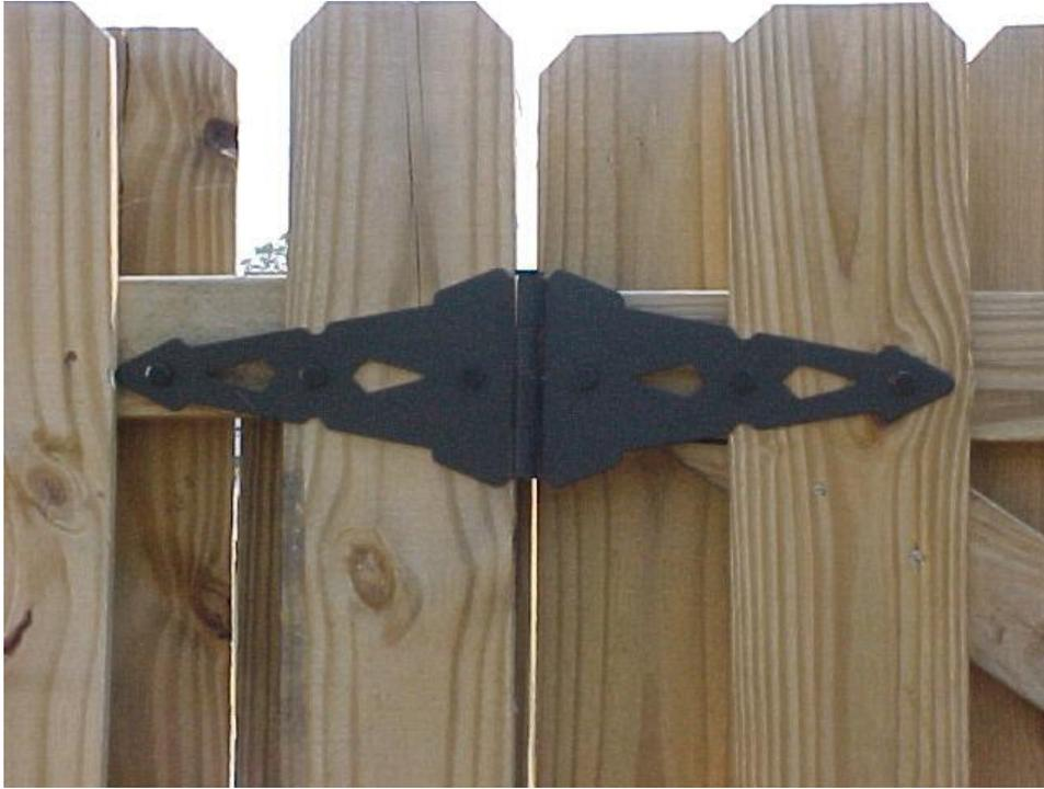
Photograph #5: Standard Gate Hinge Hardware
